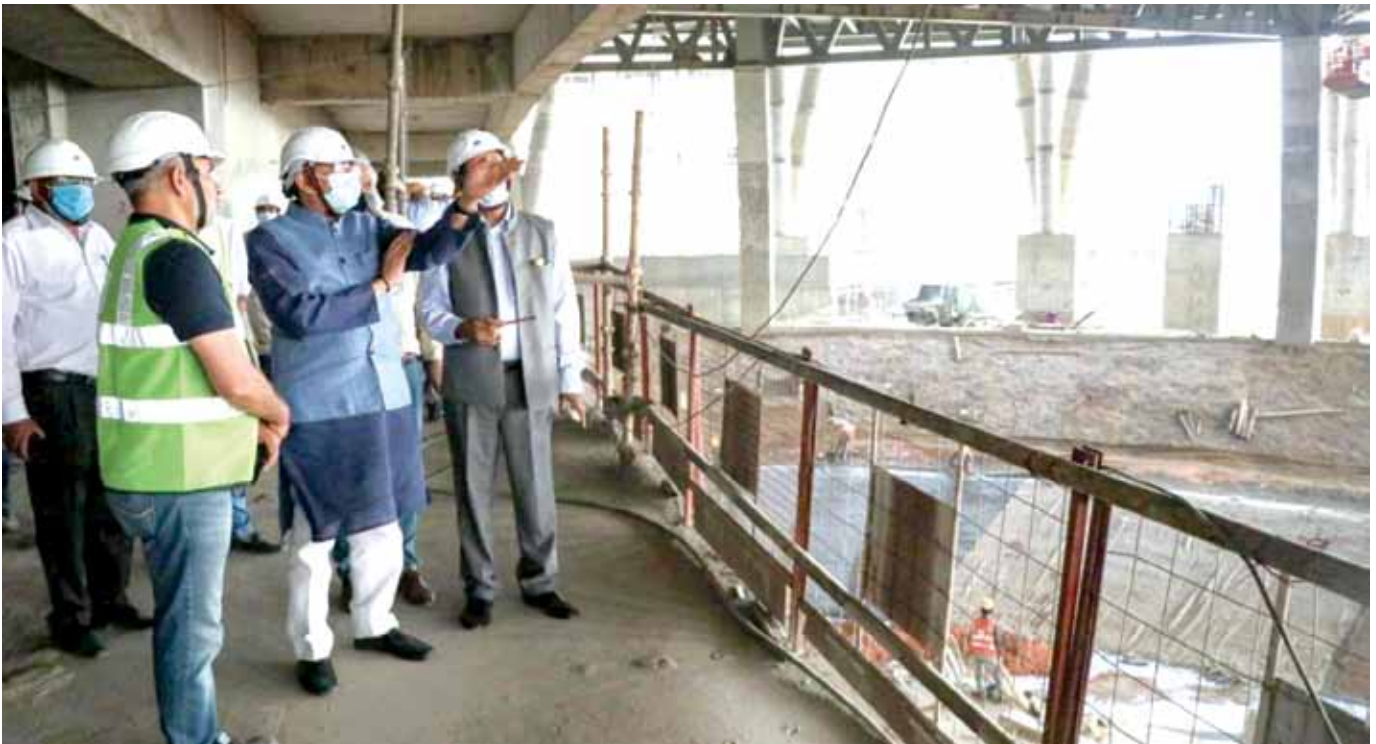
Hon'ble CIM inspecting IECC at Pragati Maidan
