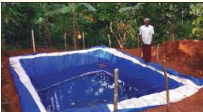
Inspection of water storage structure constructed at Rajakkad, Idukki under the scheme for Construction of Rainwater Harvesting Structure
