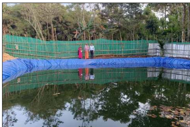
Rain water harvesting structure for small cardamom
