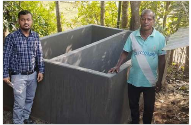
Construction of vermicompost unit in Tripura
