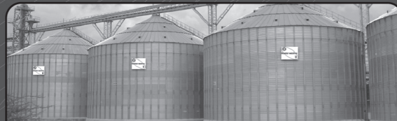
Fowler Westrup Silos
