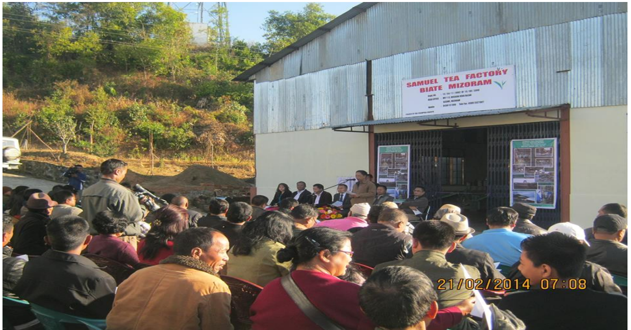
Samuel Tea Factory at Biate, Mizoram renovated / revived with the active involvement of Tea Board. Photograph taken on 21 st February 2014
